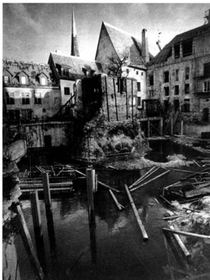
The construction crater left in the Linnateater's courtyard after the Interclub construction project was abandoned.
